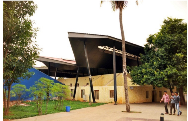
The Retrofitted “Hospital Block” [24]
